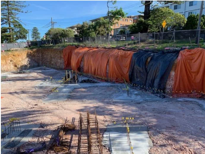
Pad and strip footings, foundation piers and lift base.
