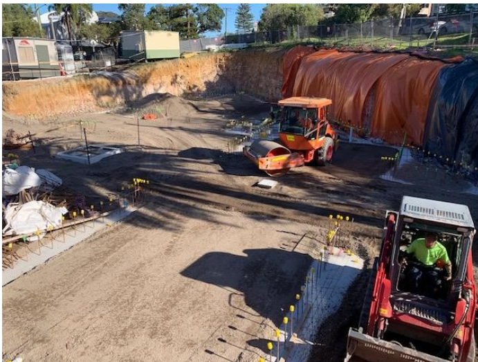
Compaction of sub-base following installation of stormwater drainage and footings.
