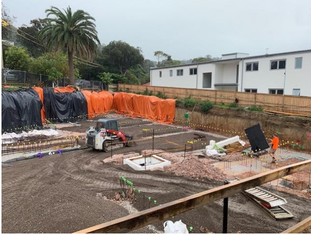
Preparation for basement slab
